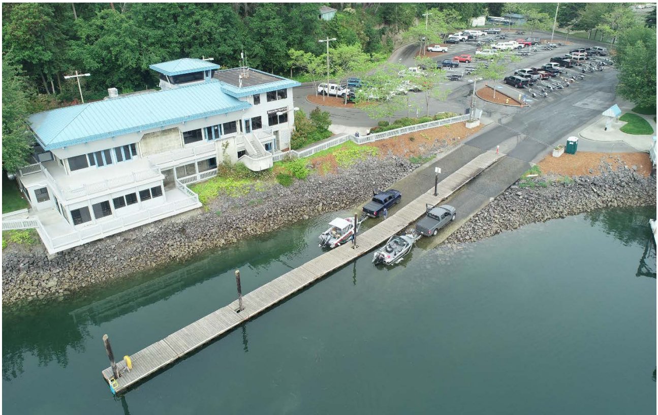
3.2_43 - JWM Boat Launch Float Replacement
