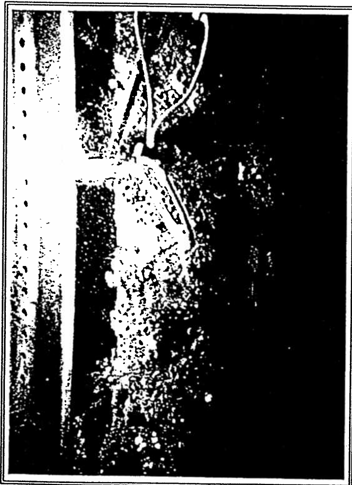
PHOTO No. 5: Mooring Float C, Pile 3 - This pile was found to have sustained a 90% marine borer cavity in the intertidal zone and has been rated in the 0% category. Note the screwdriver located in the cavity.
