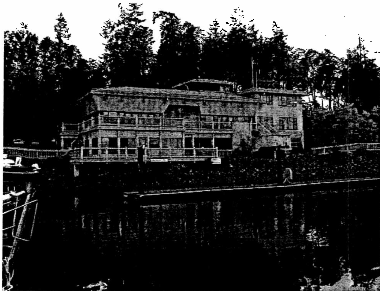
1 Harbor Master Building from boat docks
