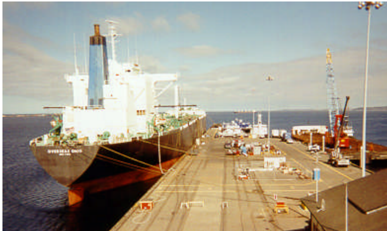
Figure 9 –Port Angeles Marine Terminal – Topside Repair
